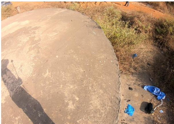
Photograph 4-7: Proposed site – existing tank bases
