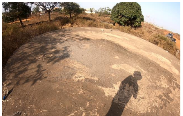
Photograph 4-8: Proposed site – existing tank bases
