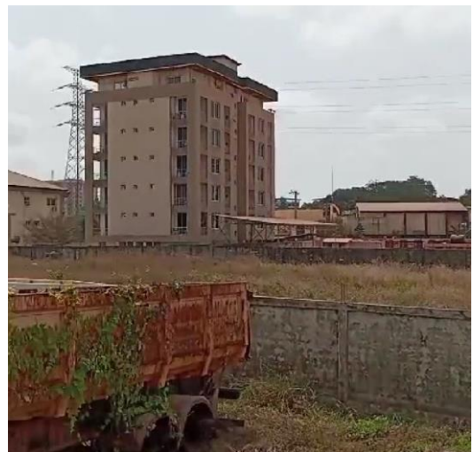
Photograph 5-4: View across site
