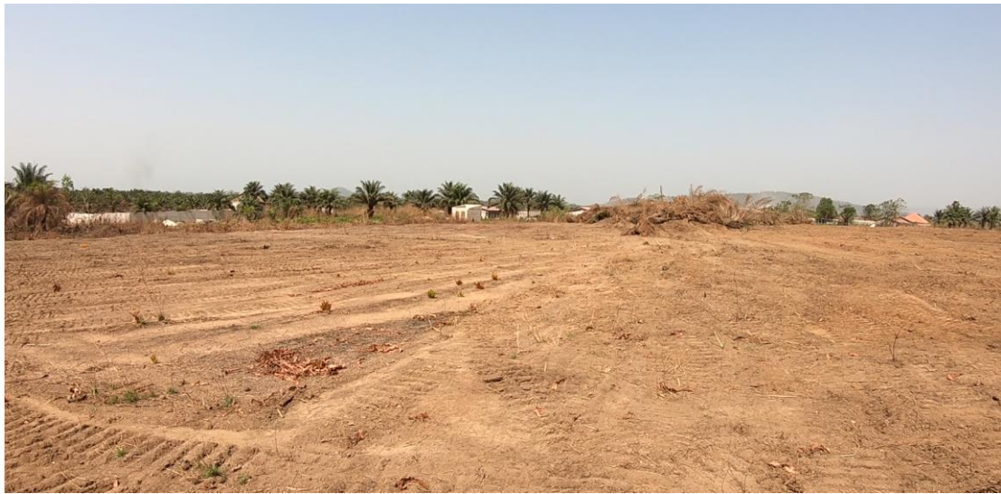
Photograph 2-4: View across Poste de Dubréka
