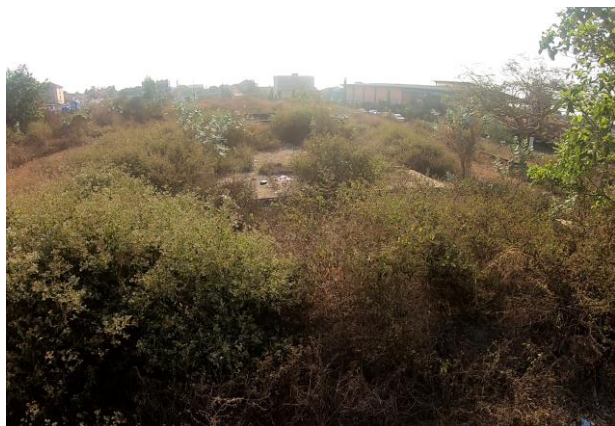
Photograph 4-9: Proposed site – existing concrete pads
