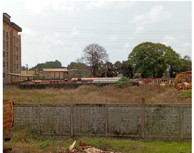
Photograph 5-2: View across site
