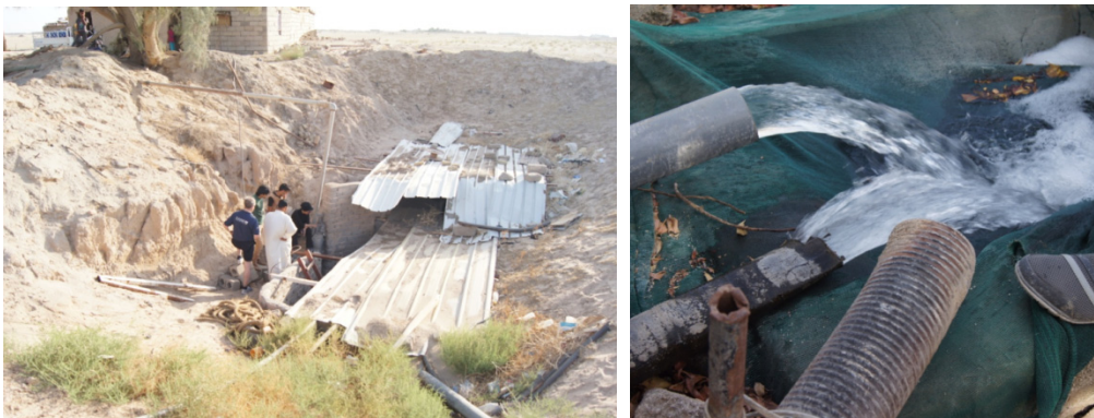
Photograph 9.1: Local groundwater abstraction (well and pump) 5km from project site
