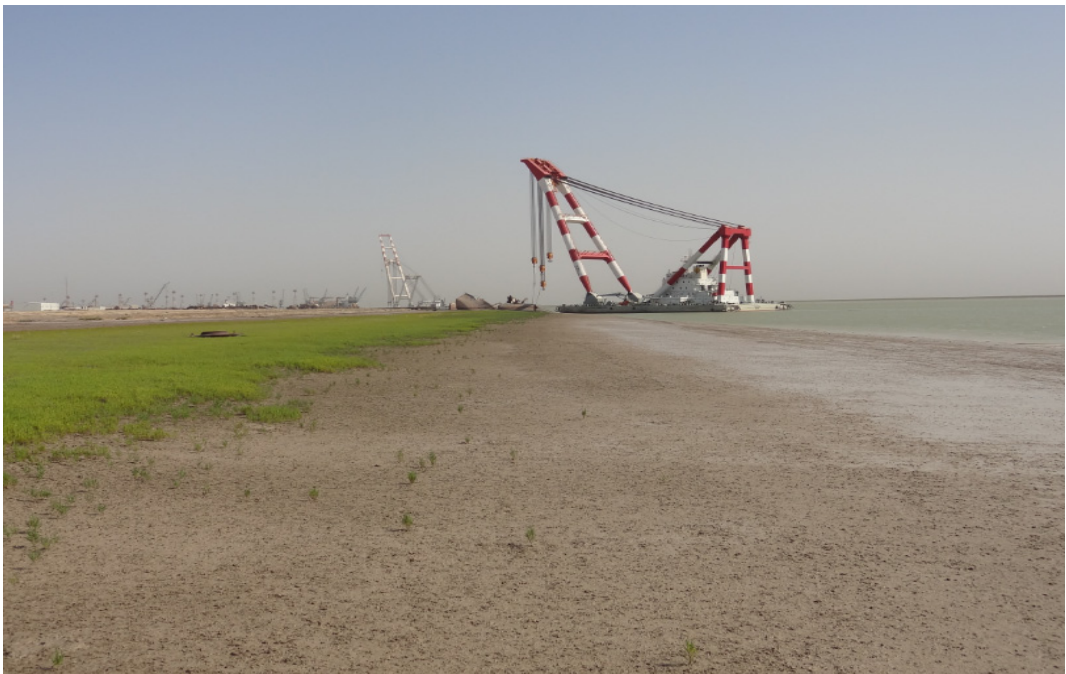
Photograph 3.6: View along foreshore towards KZP at low tide
