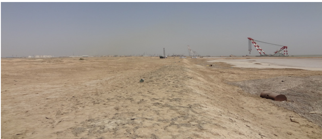
Photograph 3.4: View across the site from southern boundary
