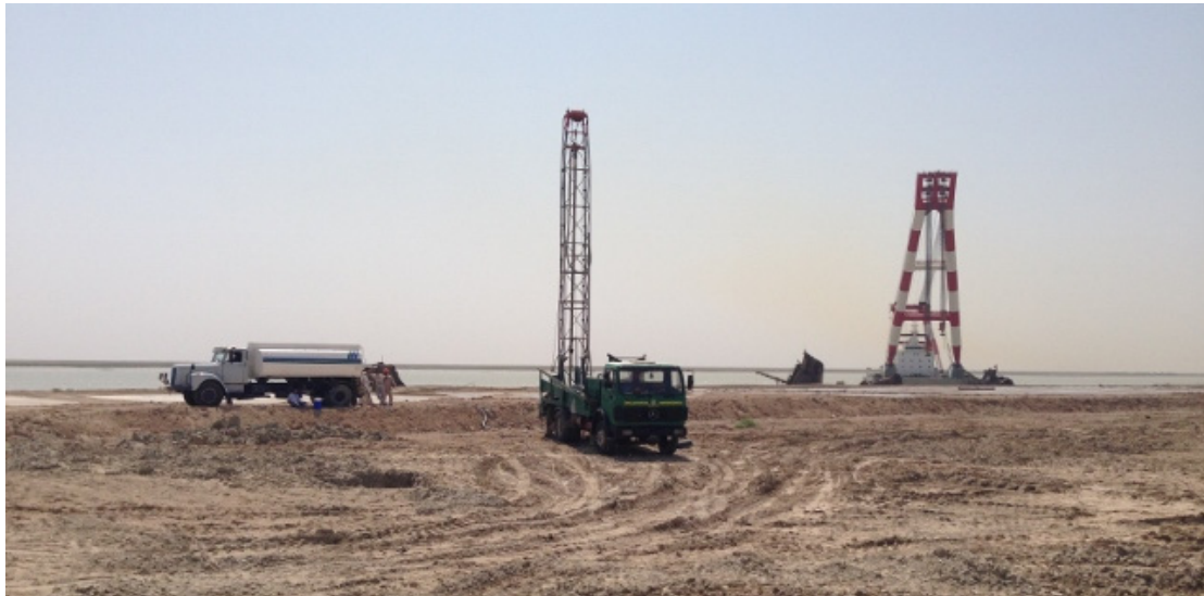
Photograph 6.1: Drilling Rig Operating BH02
