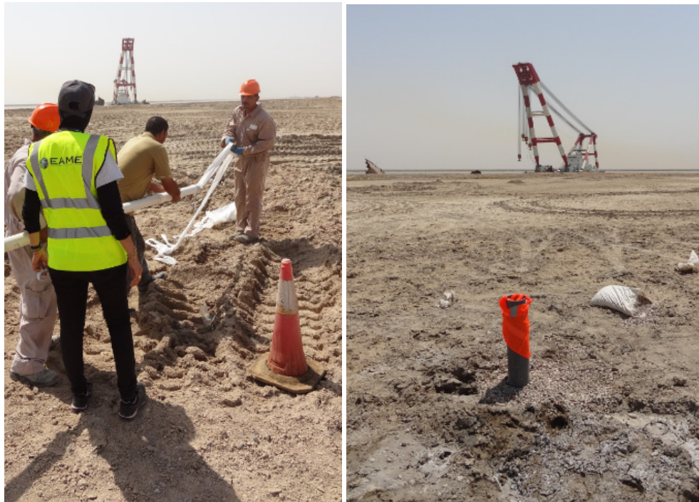
Photograph 7.1: Application of Geotextile screening sock and a completed installation
