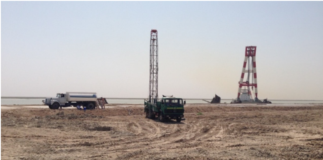
Photograph 6.1: Drilling Rig Operating BH02
