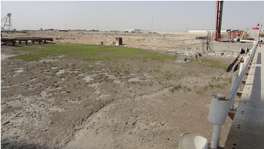
Photograph 3.7: View to the project site from KZP Berth 1
